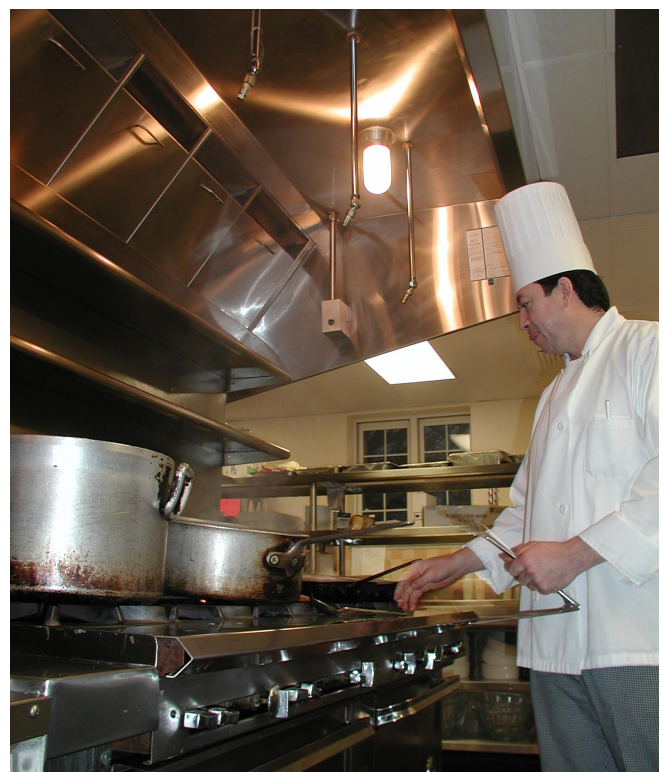
In addition to energy savings, the kitchen staff at North Shore now works in a less noisy and more comfortable kitchen, since the hood fans rarely have to "crank up" to full speed.
