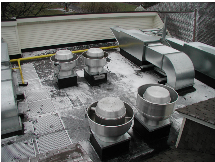
The sheer size of their kitchen operations (note the four exhaust fans in center and make-up air unit at top right) made the club a perfect candidate for the Intelli-Hood controls.
