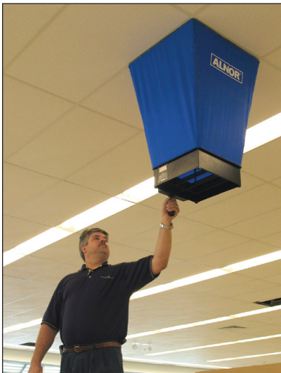
Testing and balancing in action.
