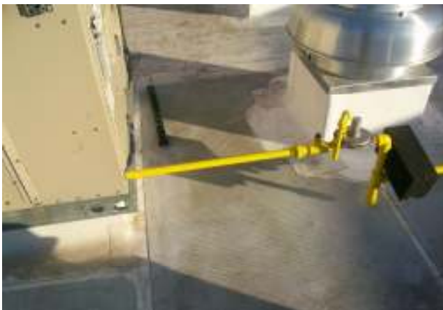
Picture 5: Gas Lines Painted
